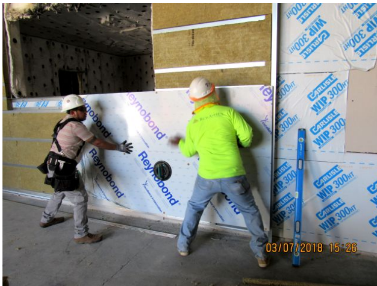
Photo No. 23 Installation of Panels
