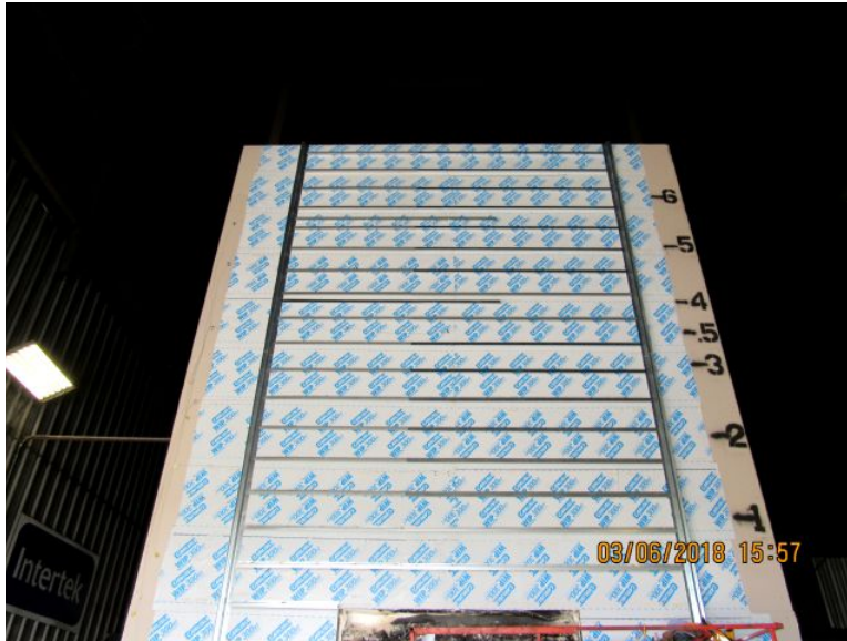
Photo No. 11 Installation of Extra Rows
