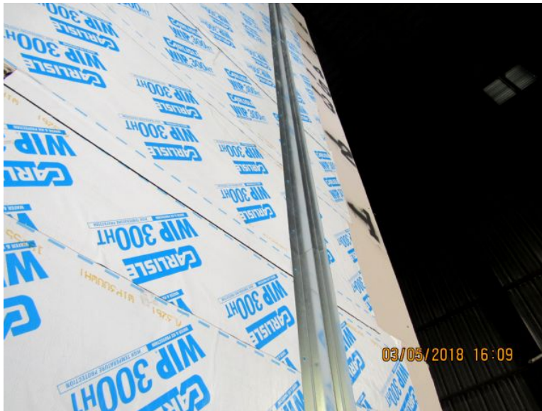
Photo No. 7 Vertical Closure
