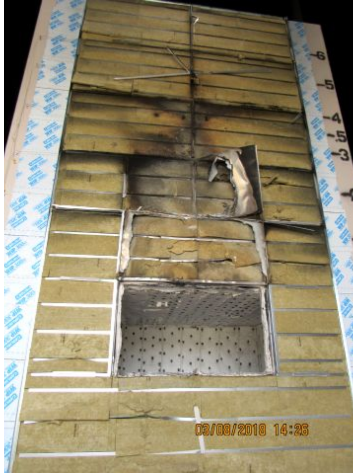
Photo No. 40 Panels Removed
