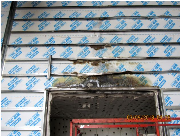
Photo No. 42 Insulation Removed
