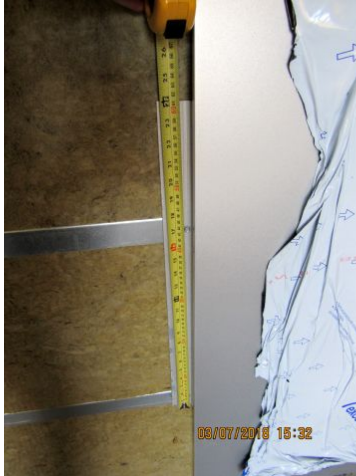
Photo No. 24 Installation of Smaller Vertical Clips
