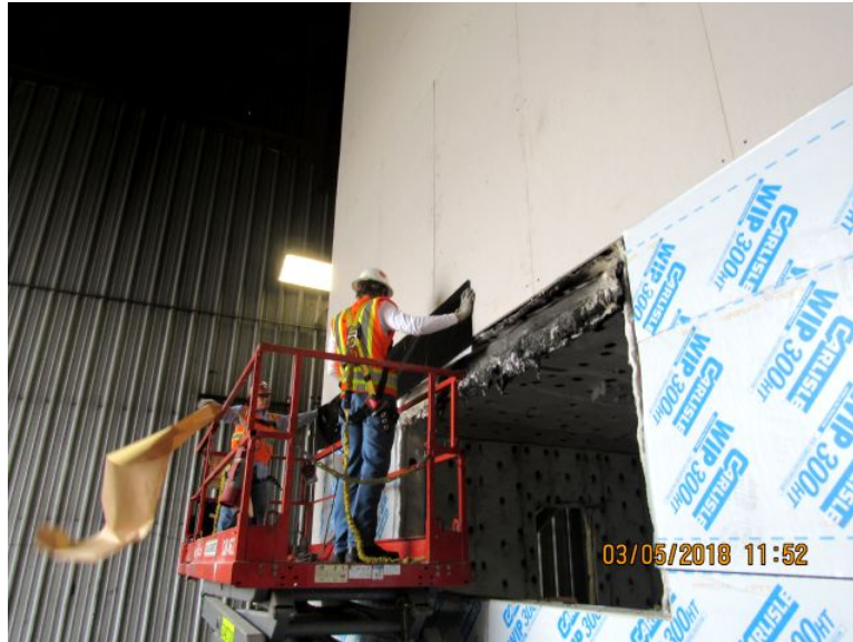
Photo No. 3 Installing Weather Barrier
