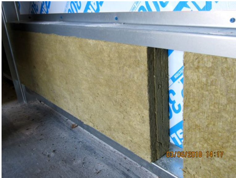
Photo No. 12 Installation of Insulation
