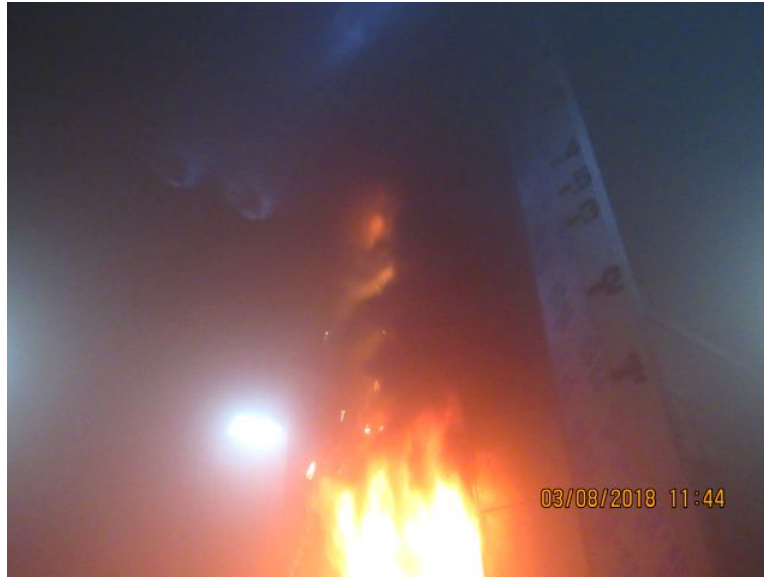
Photo No. 35 Panels Burning 4 m Above Opening
