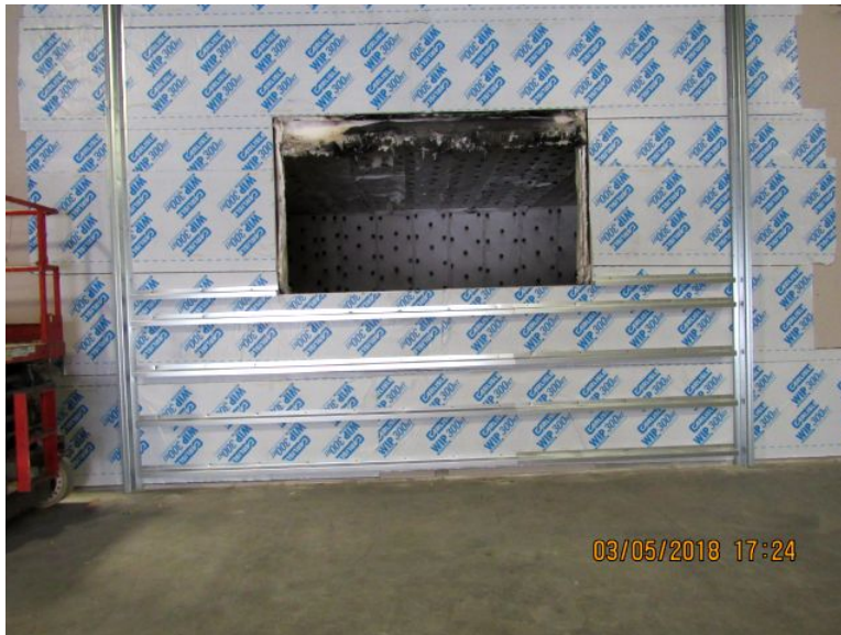
Photo No. 8 Installing Zee Girts
