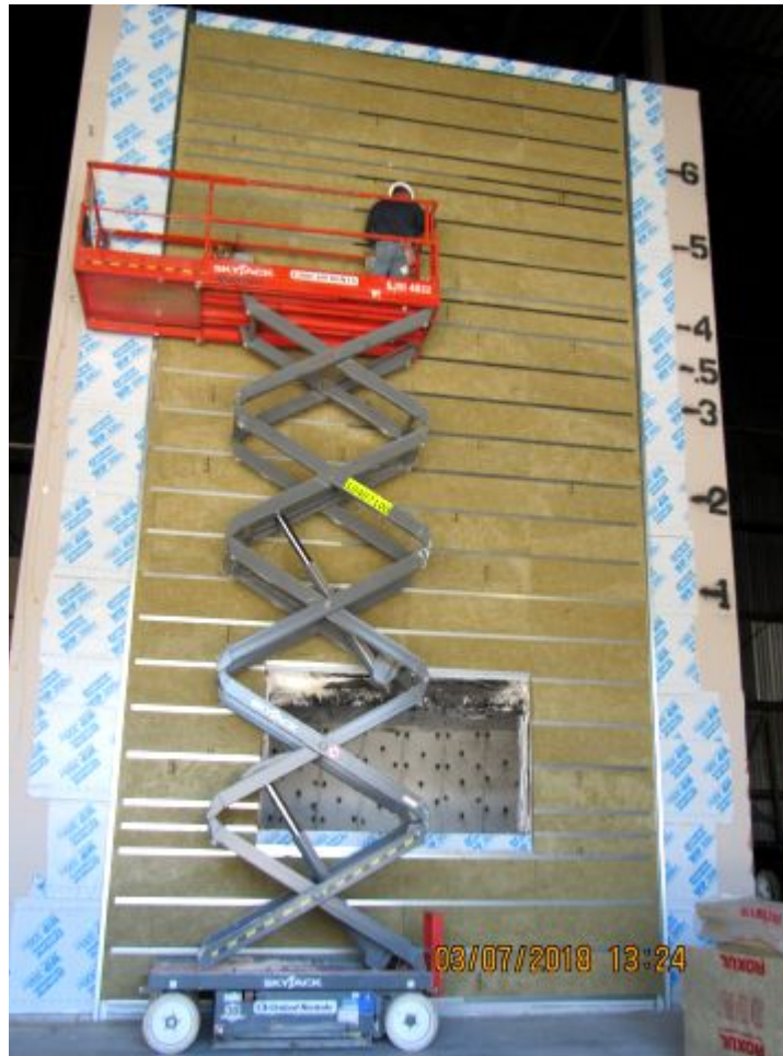
Photo No. 13 Completed Insulation
