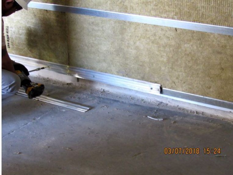
Photo No. 22 Installation of Clips
