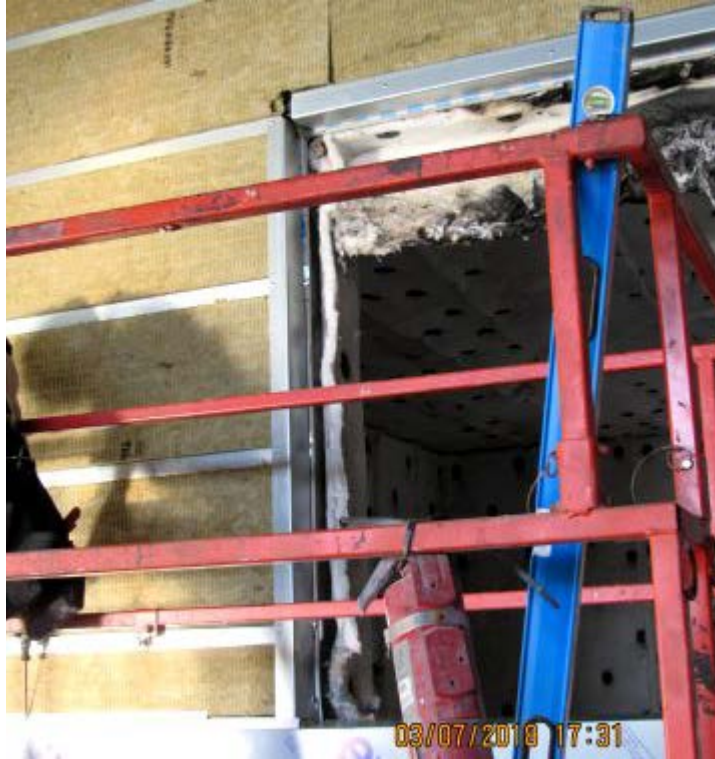
Photo No. 25 Installation of Flashing
