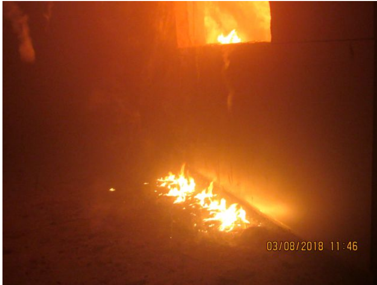
Photo No. 37 Clearer View of Fallen Debris from System
