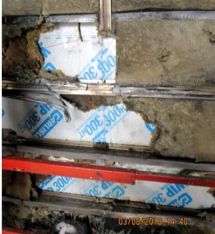
Photo No. 41 Insulation Removed Above Opening
