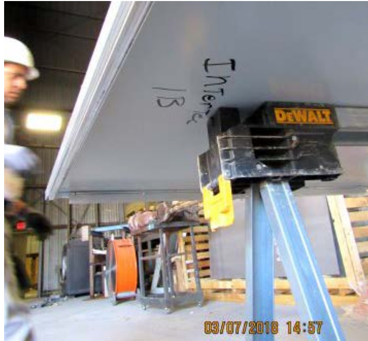
Photo No. 20 Underside Marking for Placement
