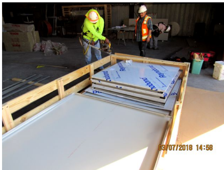
Photo No. 21 Cutting Down Middle of Clips for Vertical Edge
