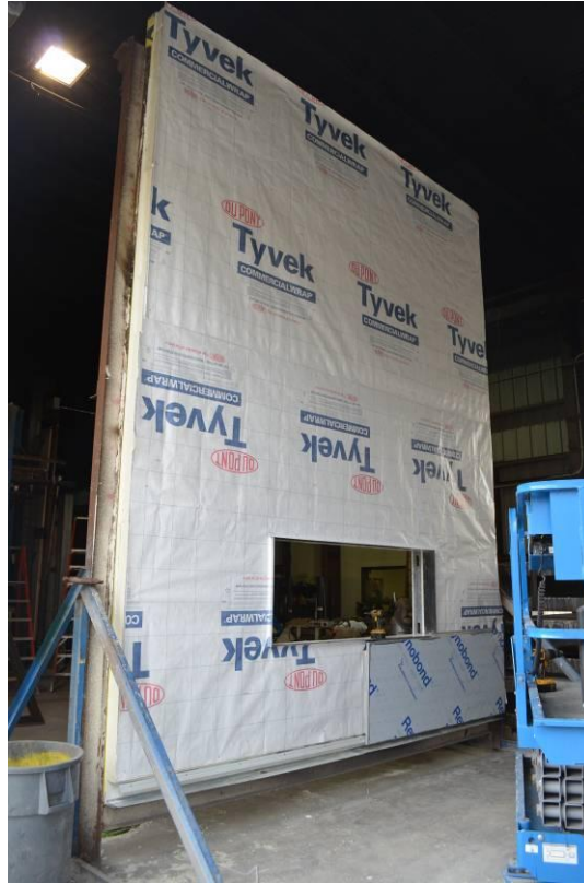
Figure B-5. Installation of DuPont™ Tyvek® Commercial Wrap over Polyisocyanurate Insulation.
