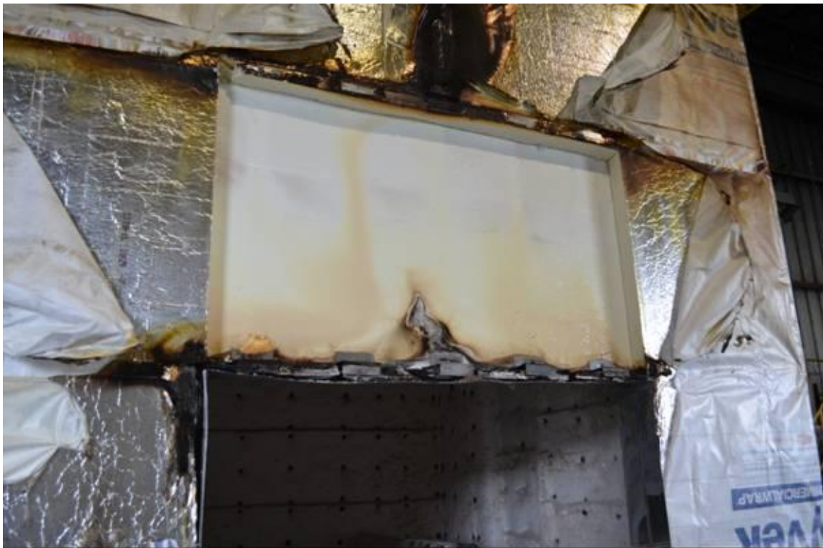
Figure B-22. Post-Test Assembly Dissection: Polyisocyanurate Insulation above Window Removed to Show Condition of Fluid Applied WB Underneath.
