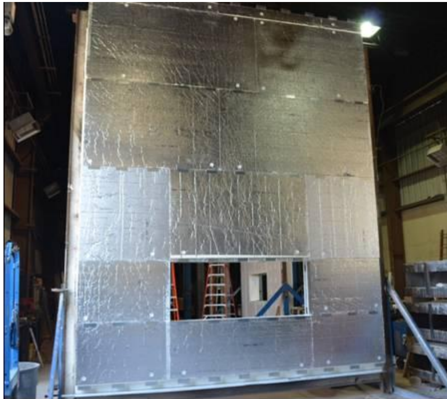
Figure B-4. Insulation installed Under Z-Girts.
