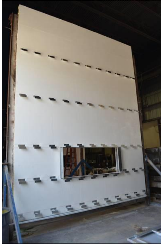
Figure B-3. Installation of Z-Girts prior to Installation of Polyisocyanurate Insulation.
