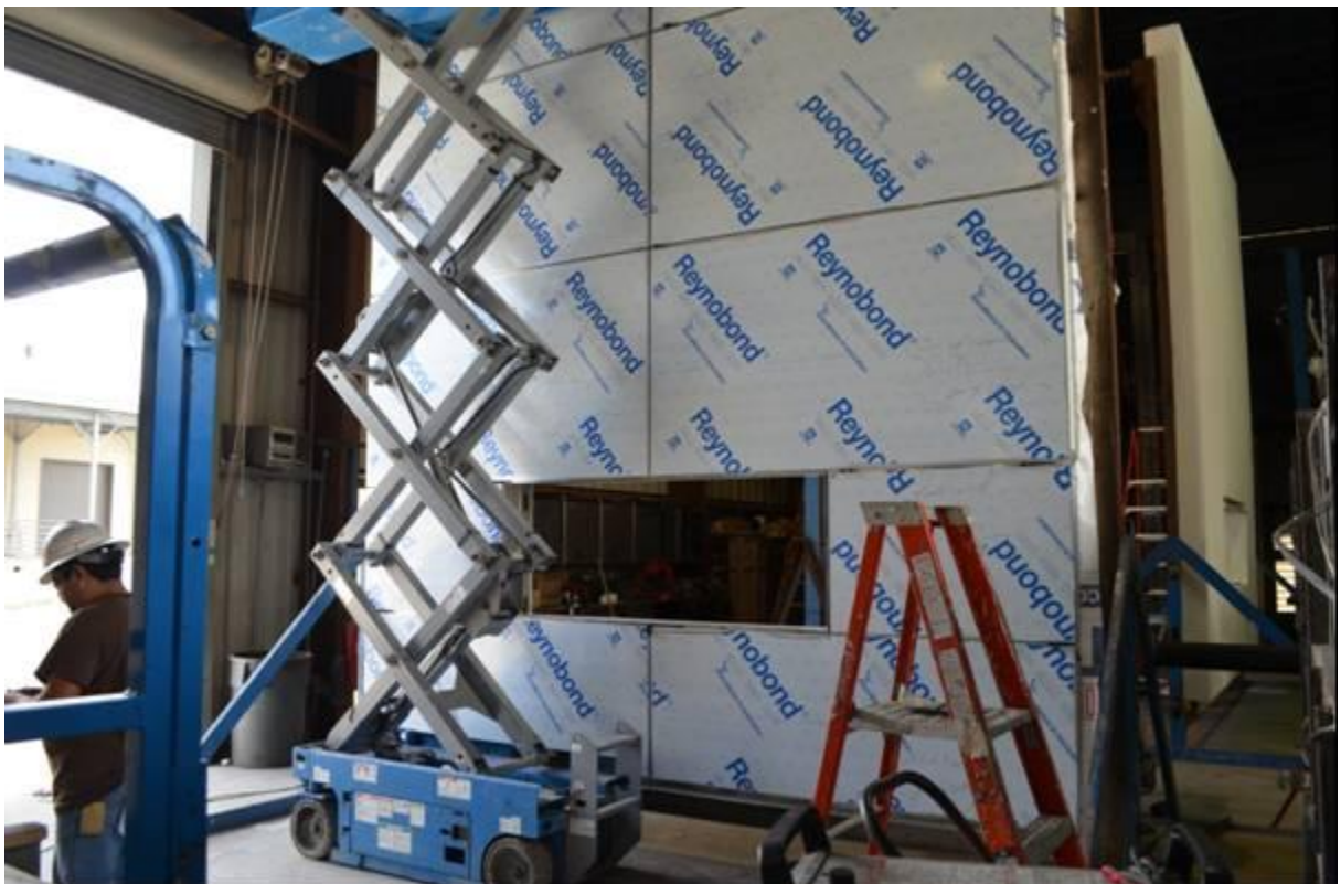
Figure B-6. Installation of Alcoa Architectural Products Reynobond 6-mm FR Panels.
