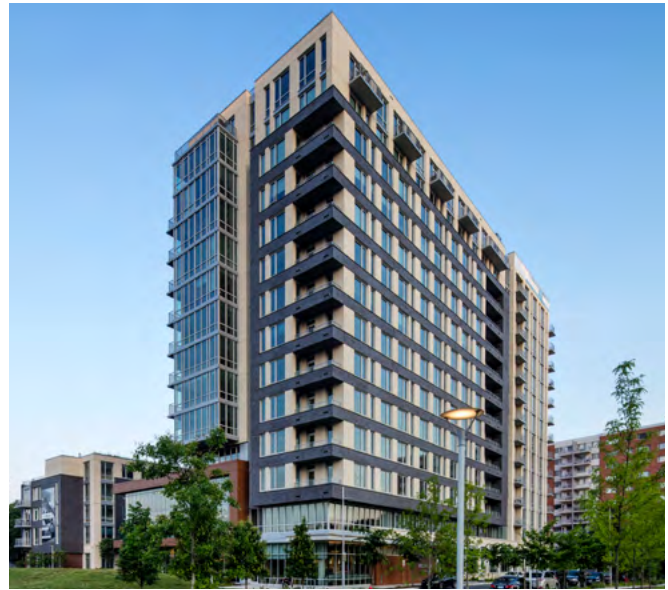
The Pearl multi-family community in Silver Spring, Maryland, comprises three buildings and features Kawneer 1600 Wall System1 and System2 Curtain Walls. The complex is LEED Gold® certified. Photo credit: Perzel Photography Group
