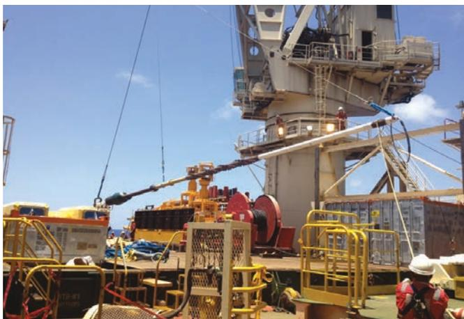
Titanium stress joint prior to installation.
